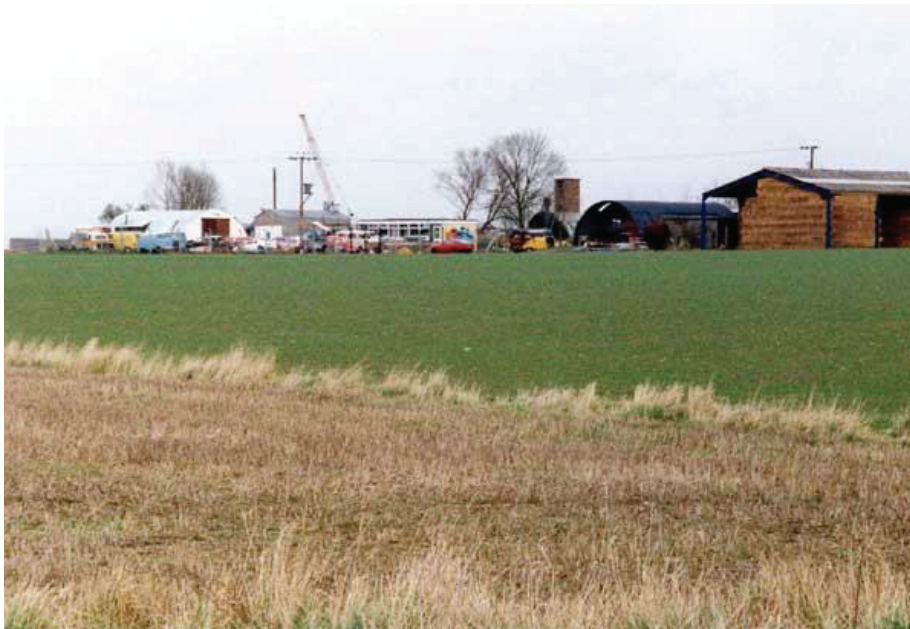
The base hospital and sick quarters were built in and around "Allshots Farm" on the South Eastern side of the airfield. Like a lot of the buildings that survive on the airfield, they have now been put to alternative use. The two dark coloured oval huts in the centre of the photo were part of the base sick quarters, each hut containing a 22 bed hospital ward.
