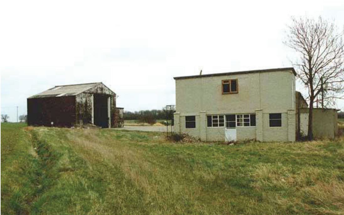
Buildings on the communal site photographed in 1996. To the left is the generator house, and to the right the gymnasium. Later when the RAF occupied the airfield this building was converted into the station cinema.
