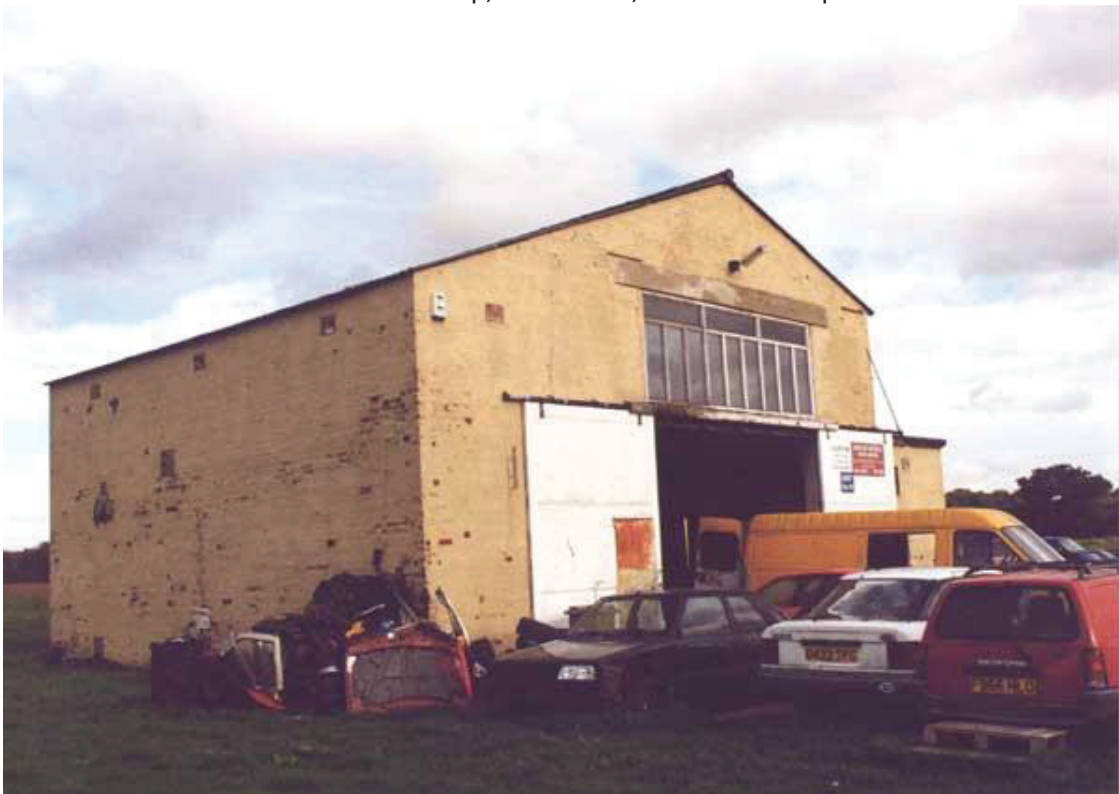
The generator house in 2001, now in use as a vehicle repair shop.
