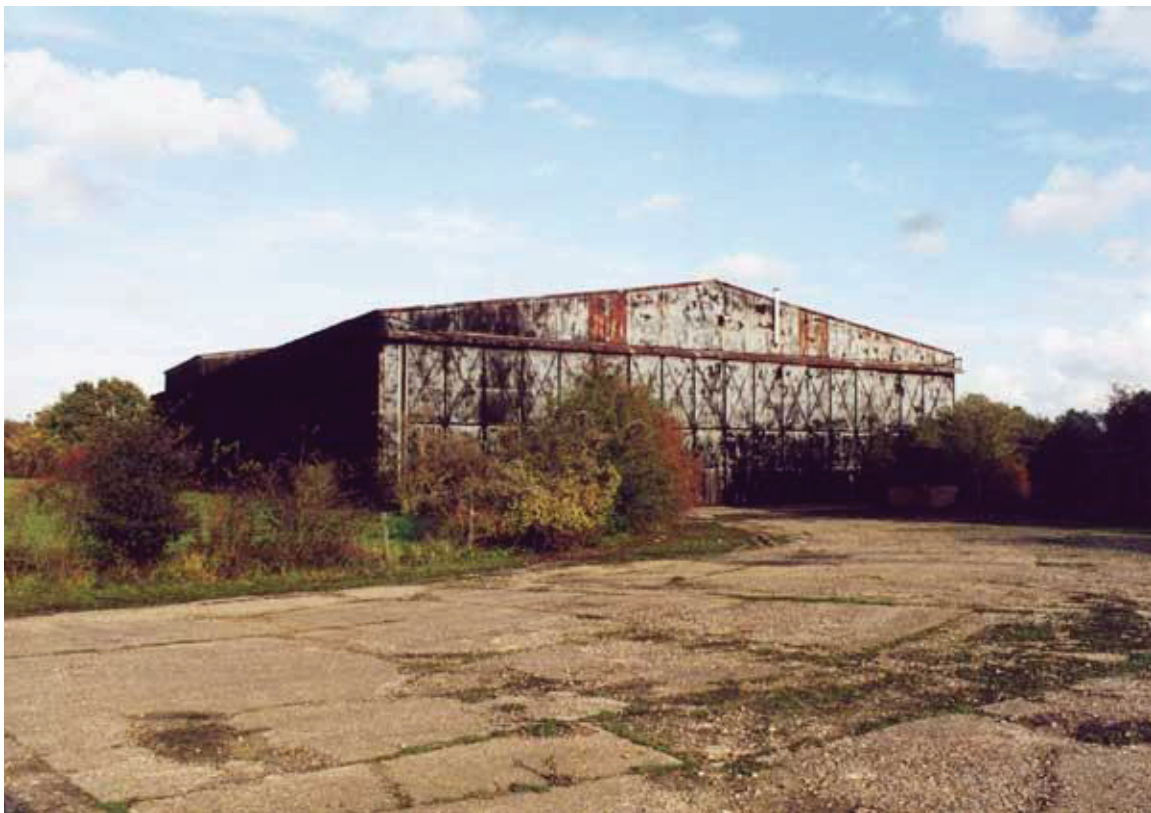
Hanger two viewed from the Southwest end.
