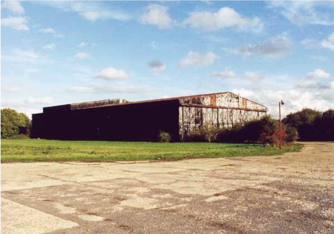
Hanger two photographed from the taxi-way. The post war altered roofline can clearly be seen from this shot.
