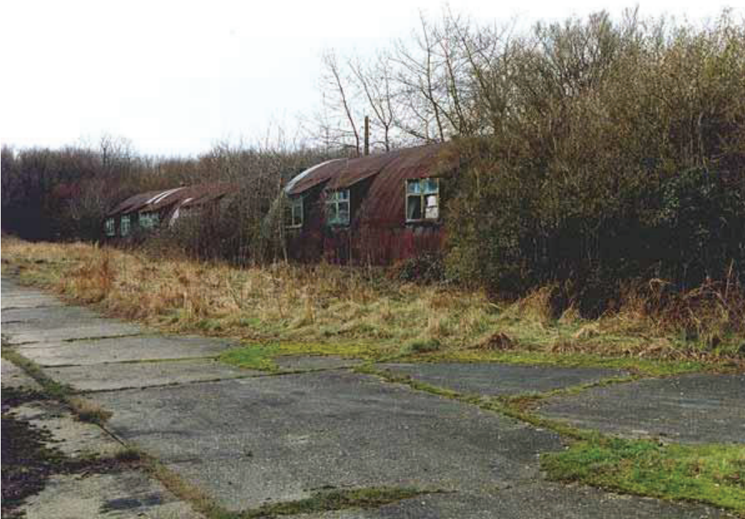
Double span Nissen huts sited to the rear of the operations block provided use as station offices
