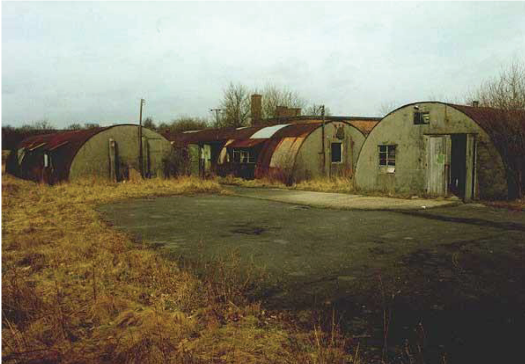
Operations buildings. From left to right, crew briefing room, office annexe, station office building. To the rear is the roofline of the base operations block
