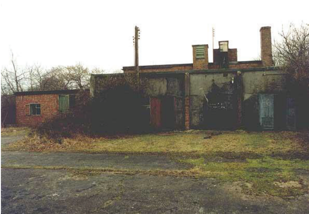
Base operations block, the nerve centre of the airfield. A windowless reinforced concrete blast proof building with its own self contained power generators and clean air ventilation system, protecting its occupants from indirect bomb blasts and the dreaded (and thankfully never implemented) poison gas attack.
