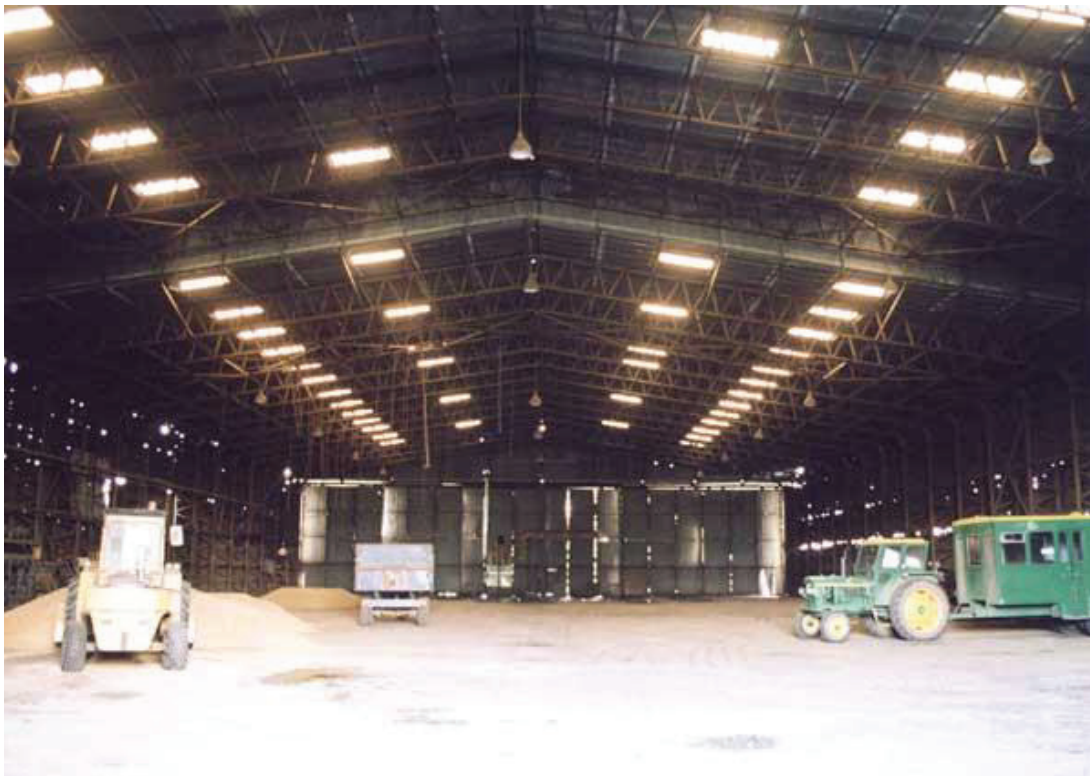
Interior shot of Hanger two. Having long since finished with aircraft servicing and repair, the building is now content to be used as a temporary grain store.
