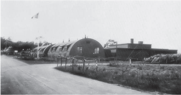
Rivenhall Airfield, England April 1944
