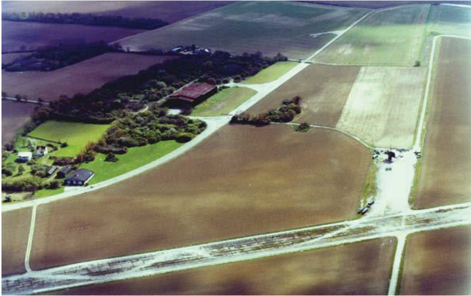
A view of the south eastern side of the airfield and hanger 1. The admin site and operations block are behind the hanger in the wooded area. The control tower was demolished after it became unstable following an explosion, but would have occupied the area now outlined by a small copse of trees almost dead centre of this shot. Note the extended roofline of hanger 1 which was converted by the "Marconi" company post war.
