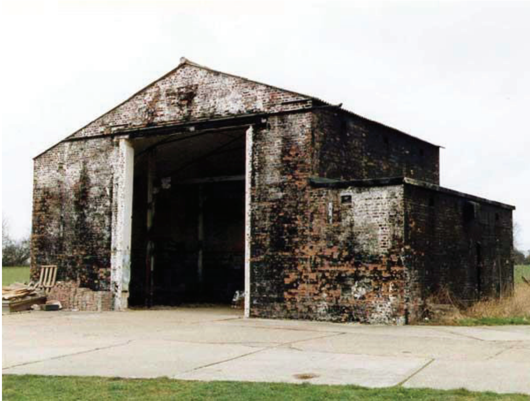
This building at the rear of the communal site was the generator house. It would have contained two electrical power generators for the base.
