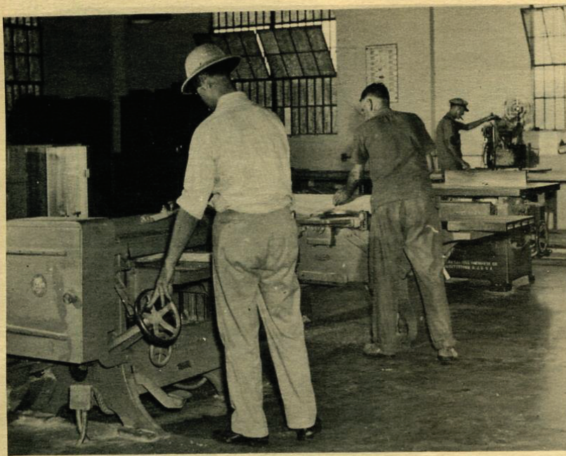
A WELL EQUIPPED CARPENTER SHOP
