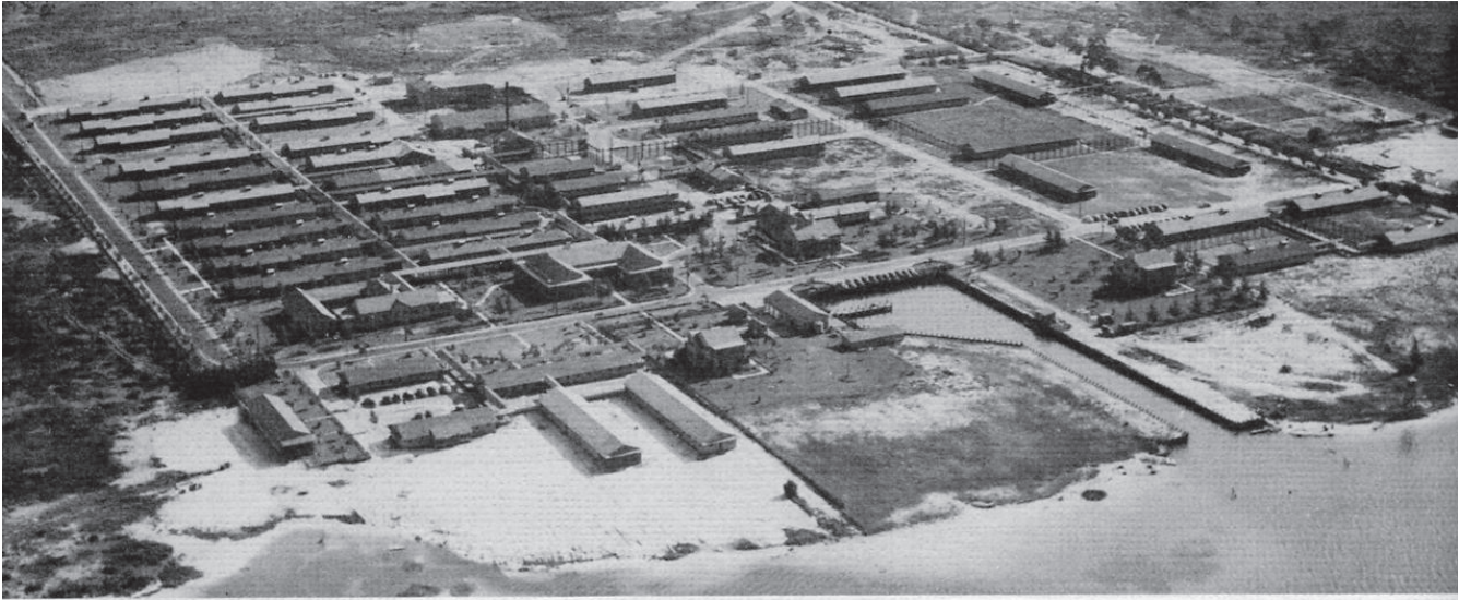
AERIAL VIEW OF MacDILL STATION HOSPITAL
