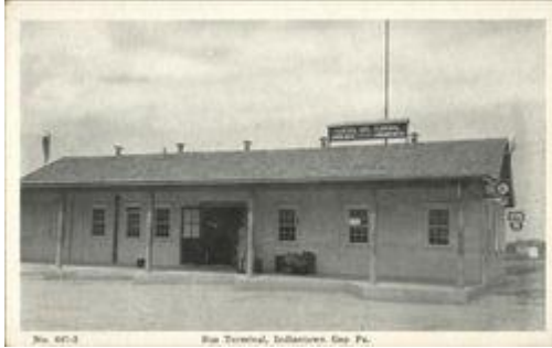
No. 67-3 Bus Terminal, Indiantown Gap, Pa. Bus Terminal Indiantown Gap Pennsylvania (PA), Linen unused
