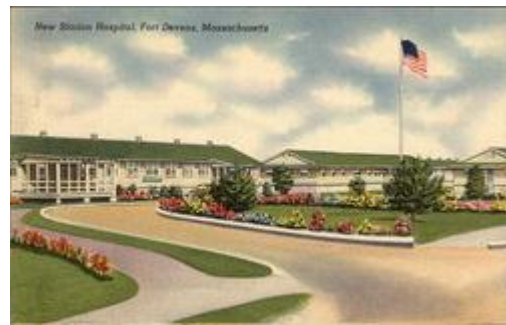
New Station Hospital Fort Devens Massachusetts (MA), Linen unused
