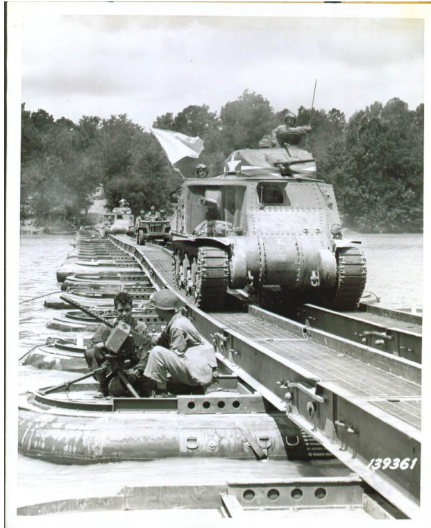
Fortified pontoon bridge over PeeDee River..1941
