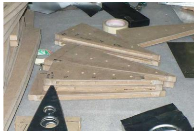
... wooden forms cut & shaped...
