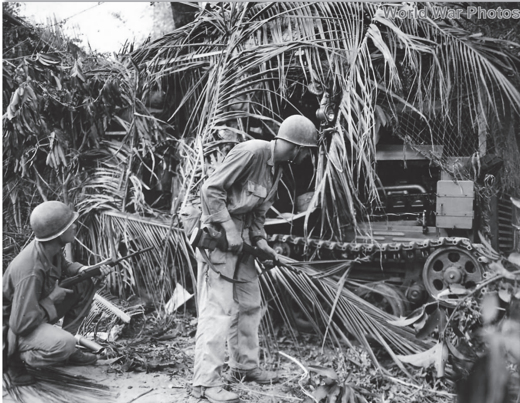
Troops Inspecting a Knocked-Out Japanese Tractor
